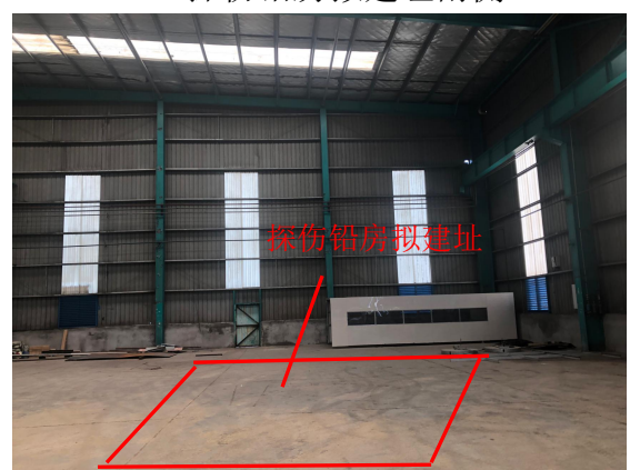
探伤铅房拟建址北侧
